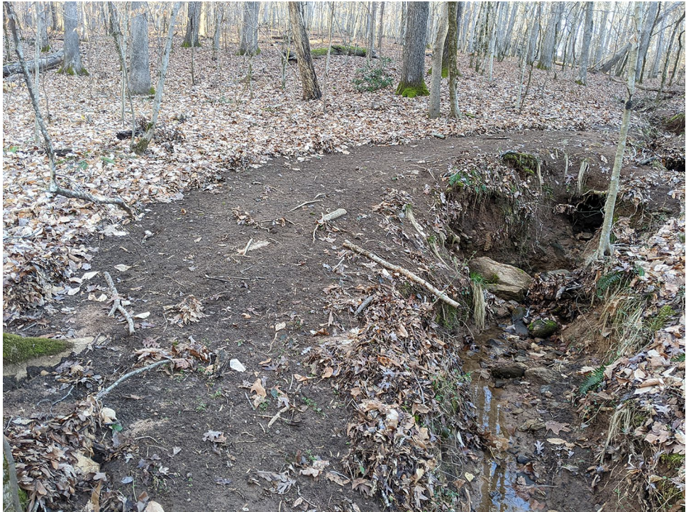
Figure 4 Bank scouring caused by winter flooding, January 2023
